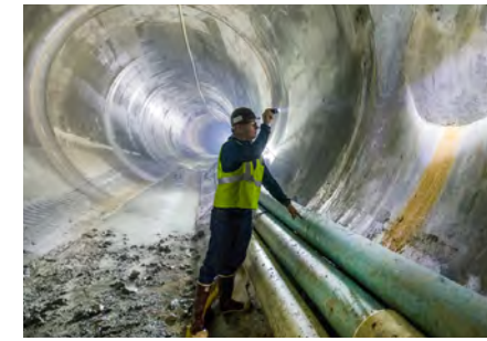
DEEP TUNNEL STORMWATER CONVEYANCE & STORAGE DigIndy, Indianapolis, Indiana
