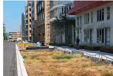
GI INTEGRATED STORMWATER SYSTEM Swale on Yale, Seattle, Washington
