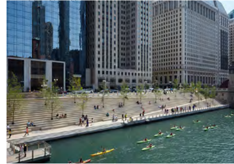
FLOOD PROTECTIONS INTEGRATED WITH PUBLIC INFRASTRUCTURE Chicago Riverwalk
